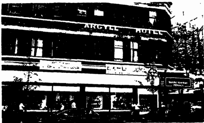
Figure 2. A Vancouver residential hotel which evicted long-term tenants to renovate rooms for Expo '86 visitors.
