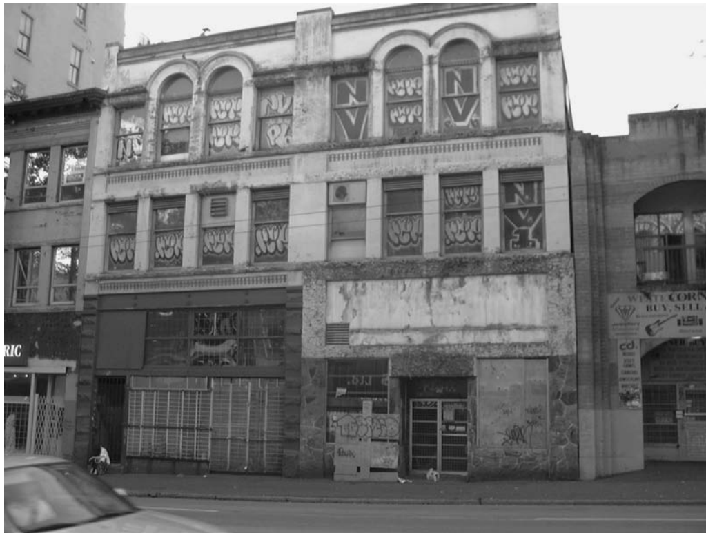
Abandoned building on Hastings Street
